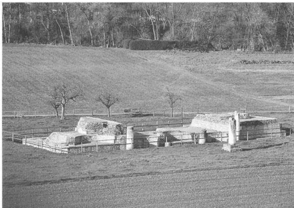
Fig. 27 Grienmatt shrine 47 , in a valley marsh to the west of the town (fig. 1, 47 ). View from the east.
