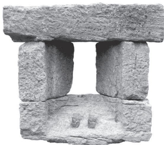
Fig. 7 Inside view of window components made of shelly limestone with mounts for a double row of bars and a shutter latch. Exterior opening 53 x 21 cm. Insula 7. Cf. fig. 8 (Morel 1991, 129, fig. 6).
